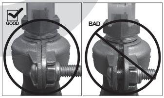
6. Visually inspect the bolt pads at each sprinkler piping connection to verify that metal-to-metal contact is achieved in accordance with step 5.
