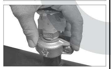
4. ASSEMBLE JOINT: Assemble the joint by installing the Style V9 onto the sprinkler piping's grooved end until contact with the center leg of the gasket occurs. Rotate the Style V9 to verify that the gasket is seated properly on the sprinkler piping's grooved end, then align the sprinkler frame arms and Style V9's bolts pads with the sprinkler piping, as shown above. A visual check is required to verify that the keys of the Style V9 align with the groove in the sprinkler piping.
