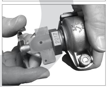
9. INSTALL NEW SPRINKLER: Insert a new sprinkler that is the proper model, style, orifice size, temperature rating, and response into the corresponding opening of the Style V9 housings. Rotate the sprinkler so that the frame arms align with the bolt pads, as shown above.
